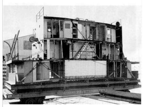
Liberty ships are famous for their all-welded construction, extensive use of prefabrication and the application of production-line techniques to shipbuilding. Above we
