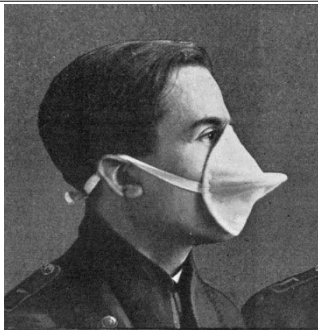
Early French design. Flannel is soaked in a chemical solution
